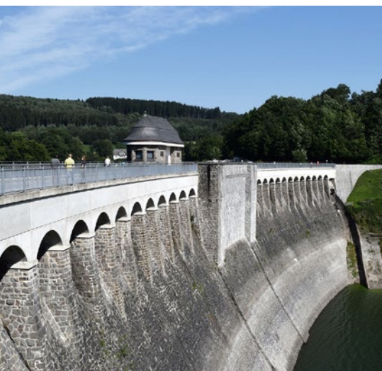
Reservoirs are often a starting point for sedimentation.
