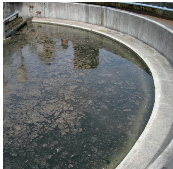
Plastics in the wastewater treatment plant after a heavy rain event
